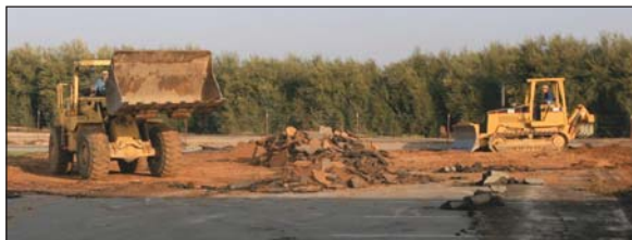
B-K Lighting North lot begins leveling for new 52,000 foot addition.
