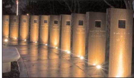
B-K Lighting provided Precision 2 HP 2 in-grade fixtures to uplight each marker for the Flight 93 Memorial in Union City, CA.
